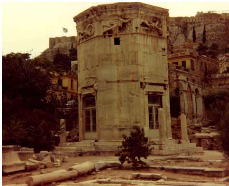
The monument of Andronicos Kyrrehestes (the “Tower of the Winds”) in Athens, decorated with eight sundials carved on the sides of the octagonal construction (north side).
